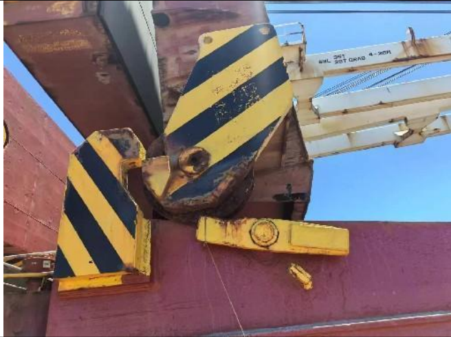
P25 hatch cover panel unable to fully open before adjustment
