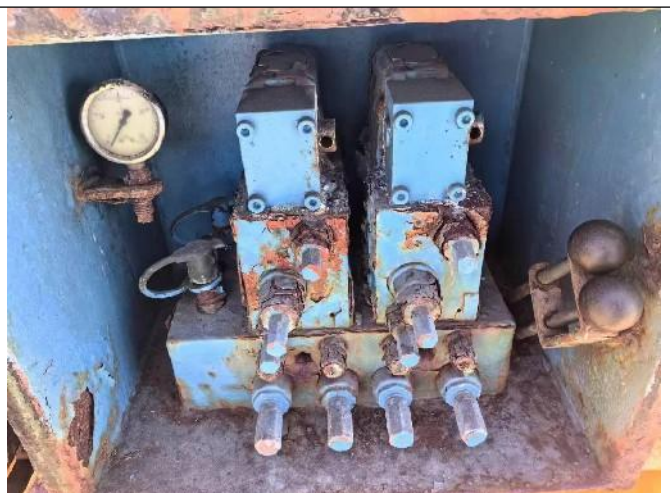
P18. Hatch cover control stand corroded
