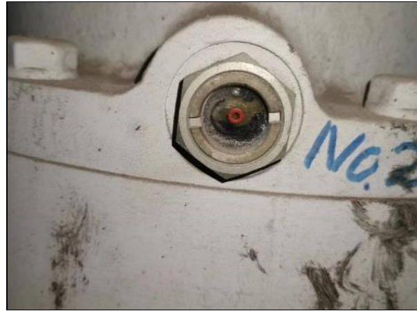
Figure 20 No.2&No.3 crane slewing gearbox oil black color
