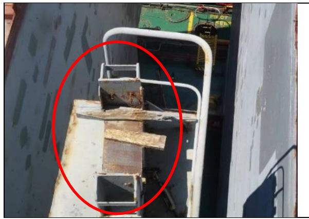
Figure 10 No.2 & No.4 crane crosser of Jib rest support lost, No.3 crane(P) support damaged
