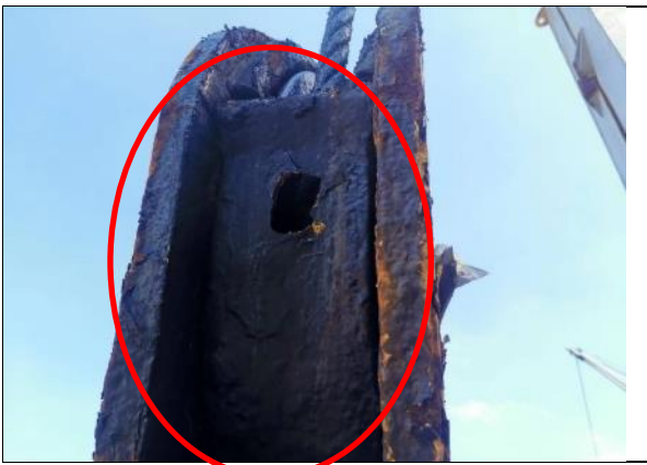
Figure 9 Hook block sheave cover corrosion badly
