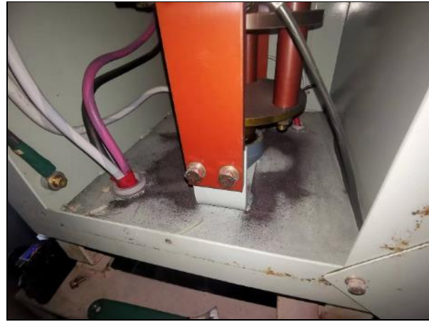
Figure 30 All crane cabin room rust (in machinery room)
