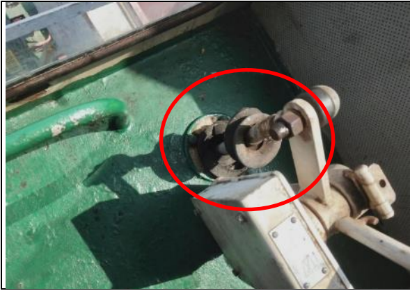
Figure 23 No.1, No.2 & No.3 crane operate handle rubber jacket broken
