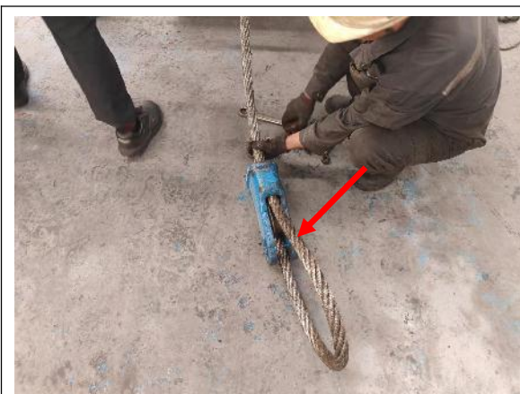
P11. wire renewed
