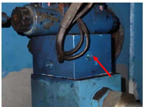
P17. valve block overhauled
