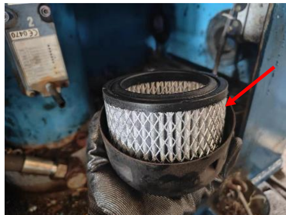
P22. air fitter had been renewed
