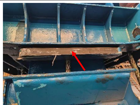
P10.rubber pad had been installed
