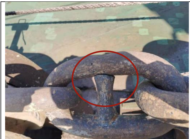
Figure 1-13 Anchor chain damaged W1
