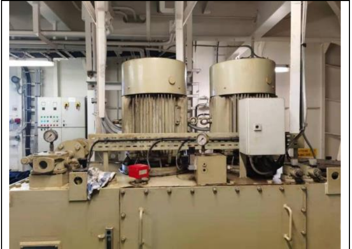
Figure 1-12 Pump station condition checked
