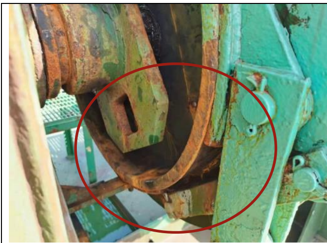
Figure 1-1 Brake lining for windlass worn out
