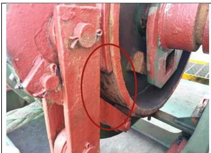
Figure 2-9 Brake lining for mooring winch worn out
